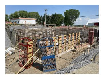
Stantec engineers selected Xypex Admix C-500, an NSF 61 approved product, to provide a permanent, integral waterproofing solution by incorporating it directly into the concrete mix for the slab and walls of both new reservoir units.
